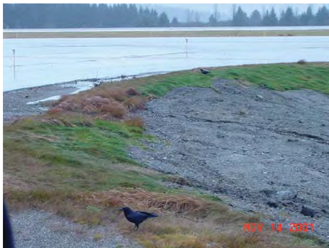
Crows attracted to fresh water trapped in berms next to a runway. These berms were caused by snow removal. (Photo E. Cleary)
