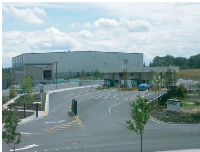
Fully enclosed trash transfer stations, such as the one shown here, generally do not attract birds. (Photo courtesy USDA)
