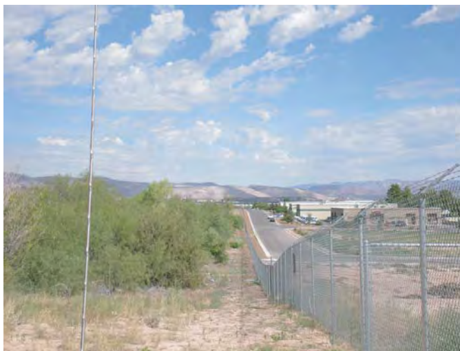
The FAA recommends a minimum 10-ft chain link fence with three strands of barbed wire for deer control. This type of fencing also greatly increases airside security. (Photo A. Dickey)
