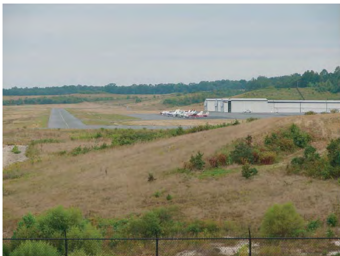
A mix of grass, brush, and trees provide near ideal habitat for many birds and mammals that can pose a threat to aircraft. Whenever possible, manage the airside vegetation to eliminate all brush and trees. (Photo E. Cleary)
