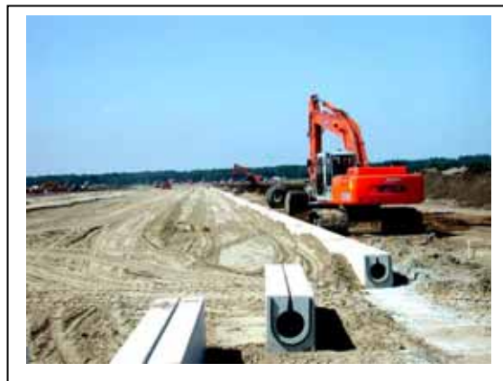
Figure 3. Slit type gutters being installed at Twenthe airbase (Photo Harrie Linckens)
