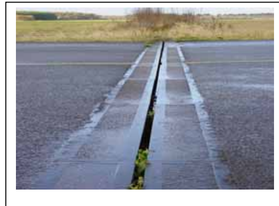
Figure 2. Slit type gutter on intersection at Soesterberg airbase
